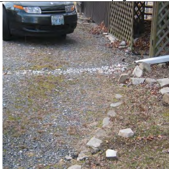
Narrow stone trench across driveway leads to rain garden on the other side
