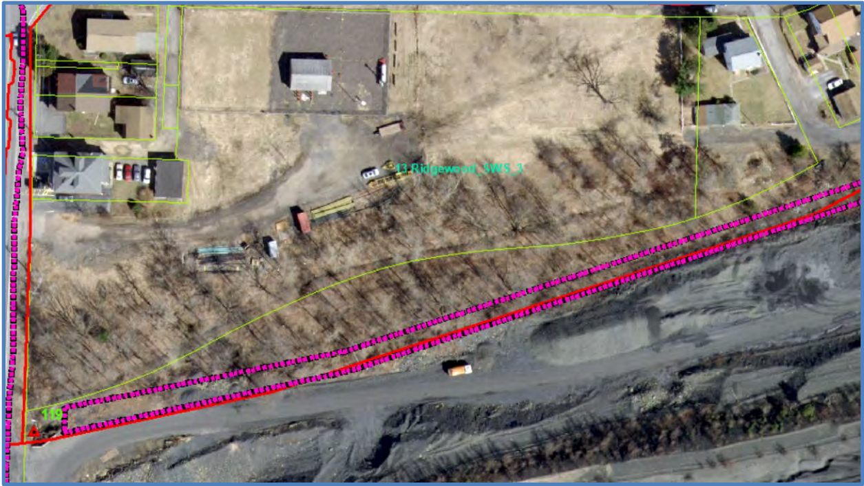
Outfall 119 - 13 Ridgewood SWS2: Outfall from conversion of old swale to infiltration swale.
