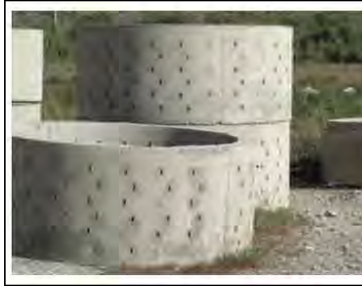
Figure E.4. Dry Well #1 – Structural Prefabricated Chamber.
